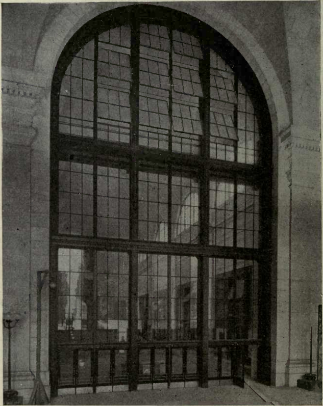
FIG. 127. — Cast-iron Entrance Screen, Pennsylvania Railroad Station, N. Y.
